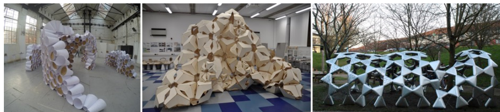
Figure 1. Element Pavilions built by First Year architecture students. Left: Perspectives Pavilion, 2018 (element: paper cone); centre: Transformer Pavilion, 2019 (element: plywood polygon); right: Seed Bomb Pavilion, 2020 (element: bent aluminium triangle).
