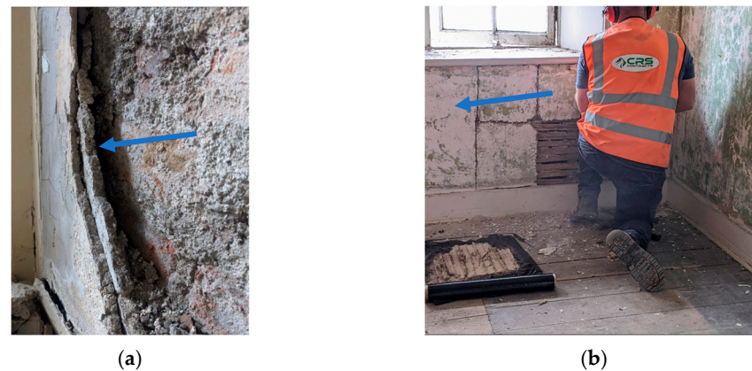
Figure 2. Plaster on a rubble stone wall during removal (a). Removal of sections of lath and plaster (b).
