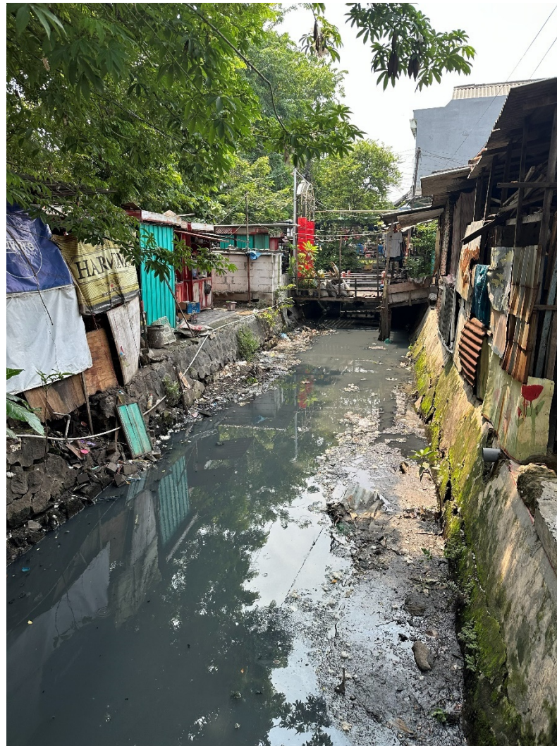
Figure 8. A view from Kampung Kue Rungkut showing its inadequate drainage conditions (photo credit: Author Iftekhar Ahmed).
