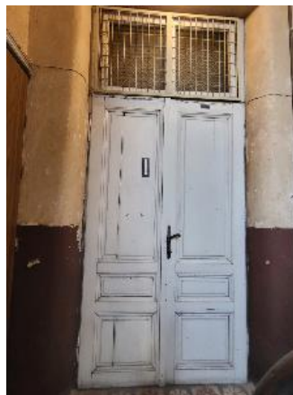
Entrance Double Doors
