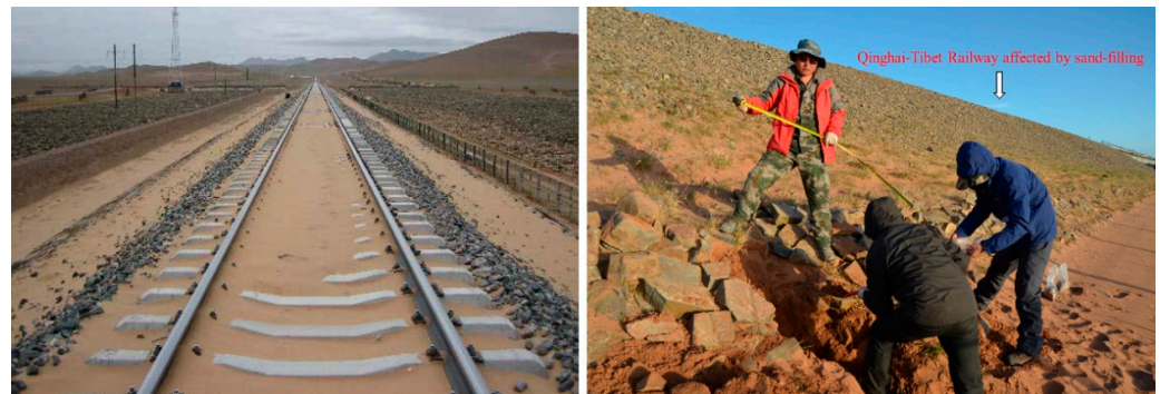
Figure 1. Qinghai–Tibet Railway affected by aeolian sand.
