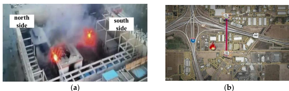
Figure 6. Fire accident at energy storage power stations: (a) Beijing; (b) Arizona.
