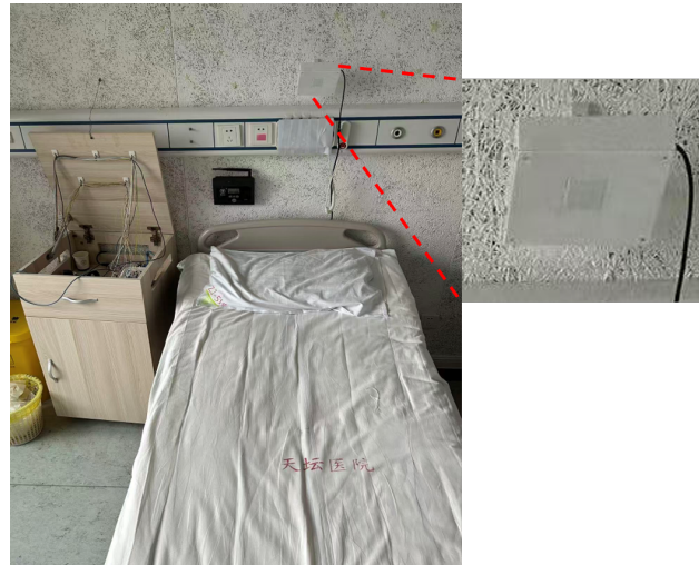
Figure 2. Photograph of the real-world data collection environment at Beijing Tiantan Hospital, showing the patient room setup and the installation position of the FMCW radar.
