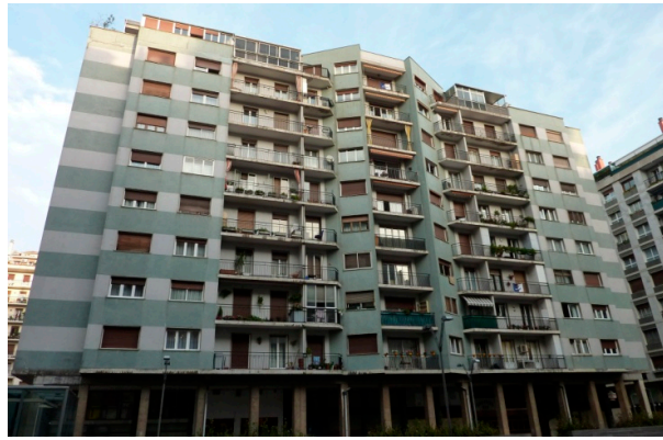
Figure 2. Picture of the case study building.
