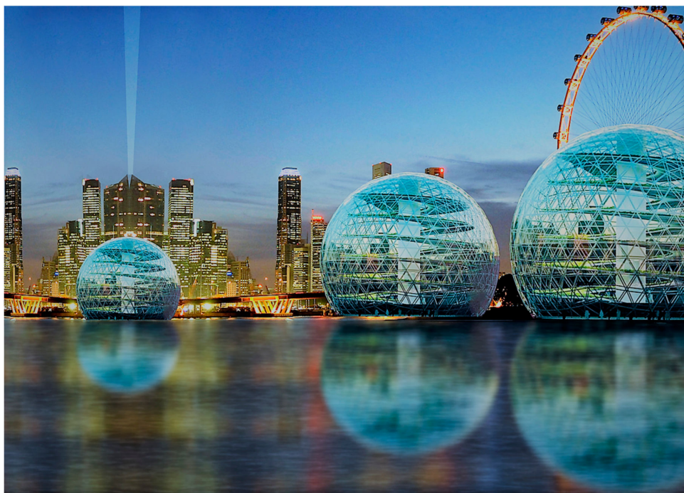
Figure 7. A proposed vertical farm by Plantagon. It comprises a helix structure placed in the center of a sphere-shaped building and stretches vertically. The helix structure contains a robot belt that instead of moving thousands of plants over the whole belt, it moves each row of plants one by one. Seeds are placed in pots on the belt at the ground floor level. Then, plants are elevated to the top by an elevator and placed on the moving belt which takes them back to the ground, and by the time they reach the ground floor, plants are ready to harvest. (Drawing by author).
