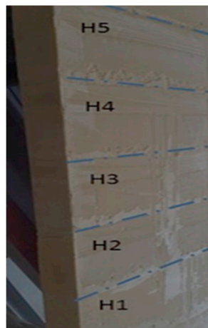
Figure 9. Casting schedule of seams at specimens with transverse seams (TS). Locations of transverse seams.
