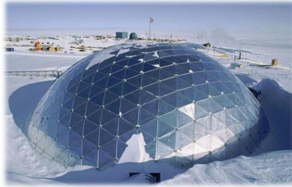
**Figure 7.** Metal geodesic dome of the US Antarctic Station Amundsen–Scott.
