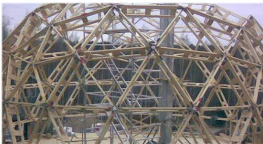
**Figure 4.** Two-layer geodesic dome structure.
