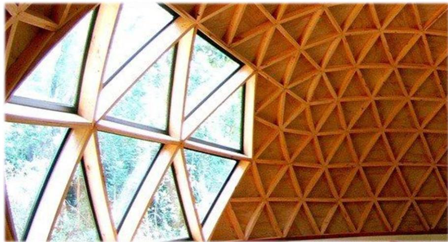
Figure 1. Single-layered dome structure without thermal insulation.
