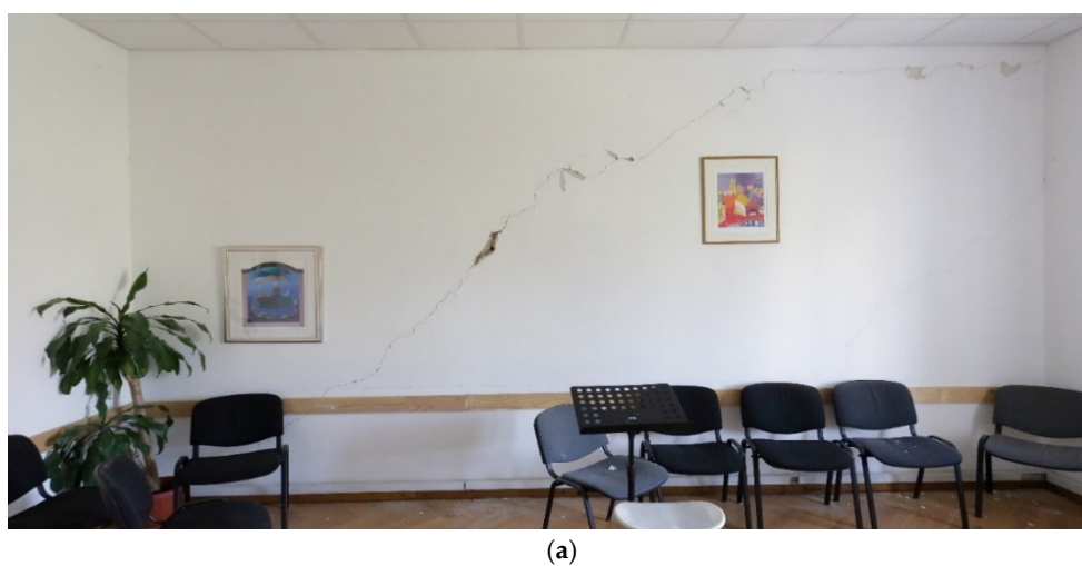
Figure 8. Diagonal X-pattern cracks on parapet walls between the first and second floor.
