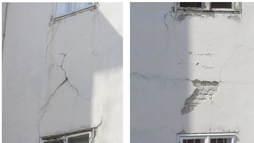
Figure 8. Diagonal X-pattern cracks on parapet walls between the first and second floor.
