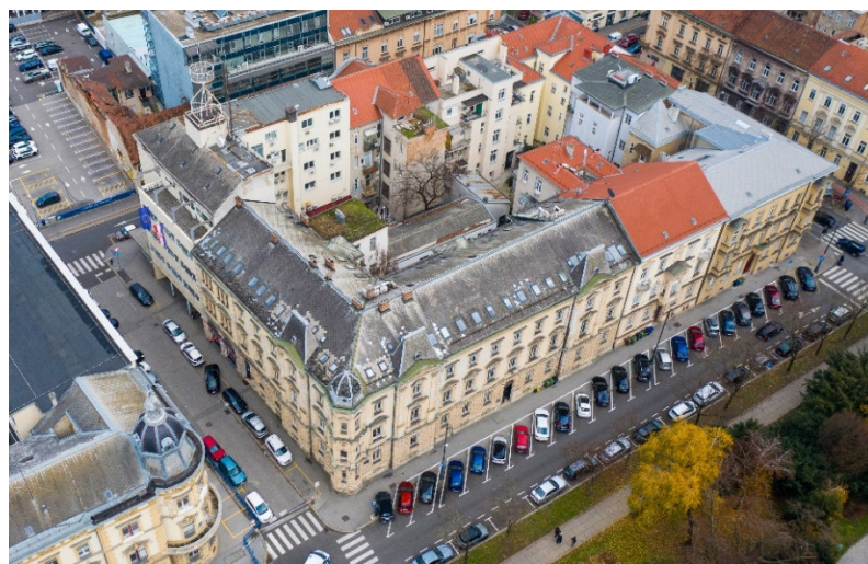
Figure 4. Aerial view of the building (photo credit: Mislav Stepinac).
