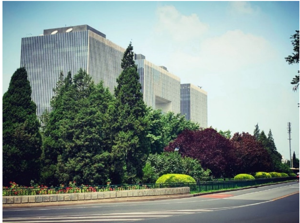
Figure 5. China Petroleum Tower (from Baidu Map).
