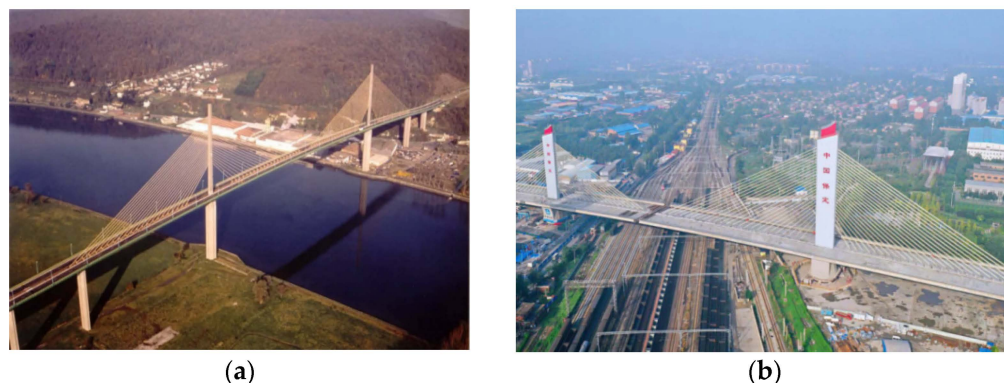
Figure 1. (a) The Sunshine Skyway bridge; (b) LeKai South Extension bridge.
