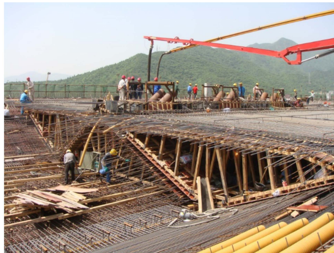
Figure 2. W-shape diagonal web section construction.
