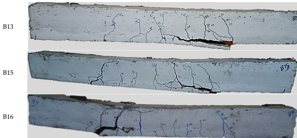
Figure 19. Mode of failure of beams B13, B15, and B16.
