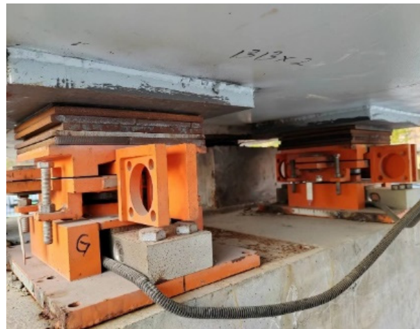
Figure 9. The intelligent force-measuring bearing.
