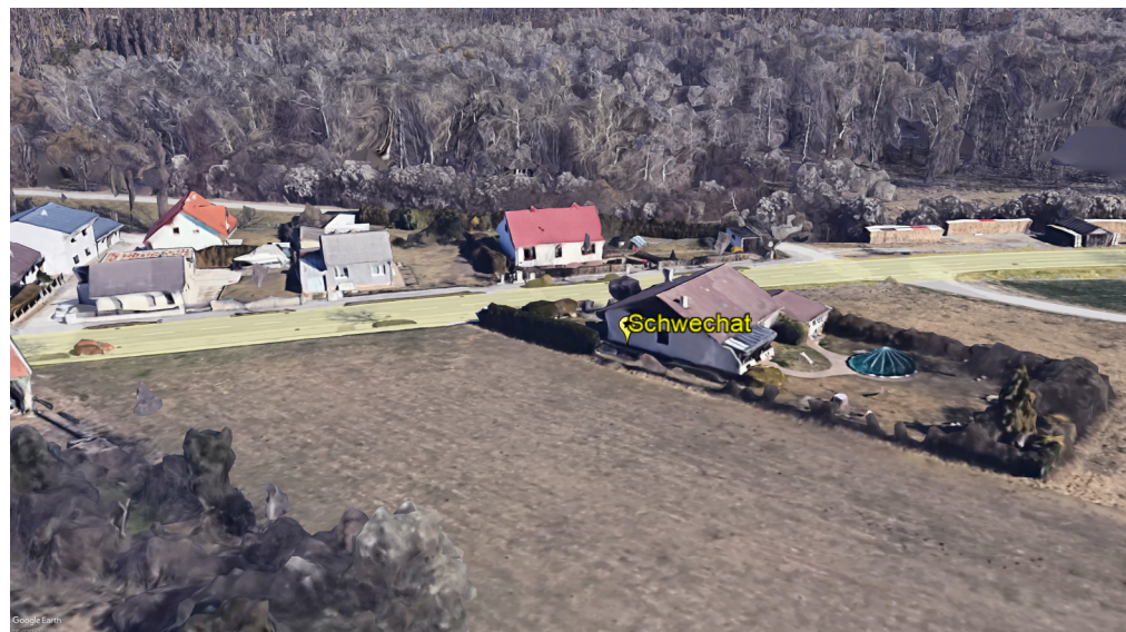
Figure 16. An individual isolated building on the city's outskirts, Schwechat region, Vienna [57].
