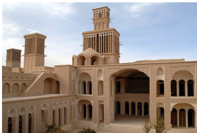
Figure 7. Multi-story windcatcher, Aghazadeh mansion, Yazd, Iran (Photo by Salehzadeh, S.) [12].
