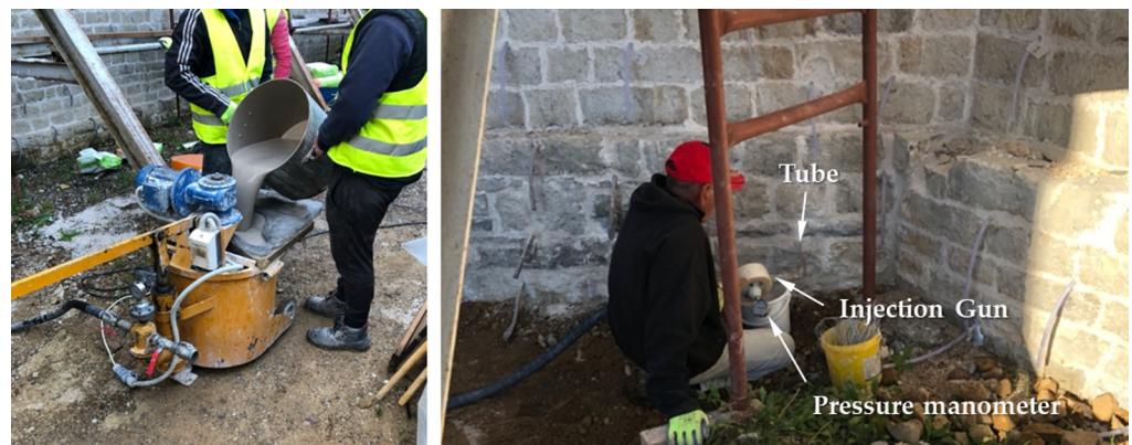
Figure 3. (Left) The mixing tank and pump with pressure manometers, where the grout was mixed with the appropriate amount of water. The mixture is filtered to remove coagulated particles. (Right) Grouting at the eastern masonry at an exterior tube position and monitoring of pressure on the manometer of the gun.
