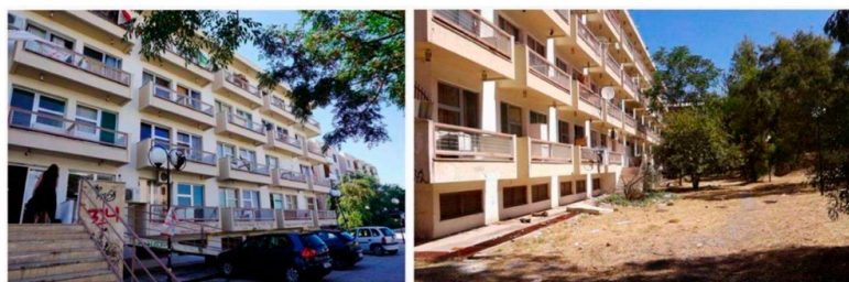
Figure 2. The student house in its pre-renovation state.
