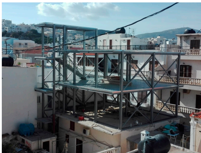
Figure 1. Mixed concrete/steel structure.
