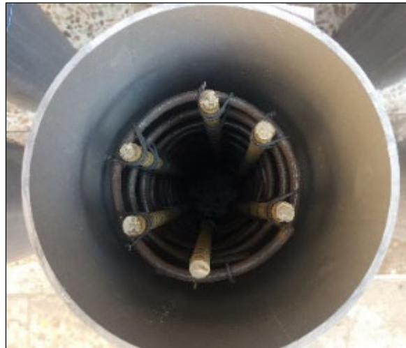
Figure 3. Reinforcements inside PVC formwork.
