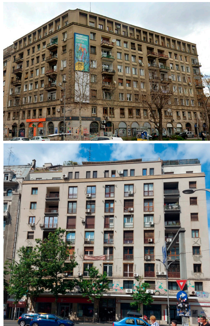
Figure 12. Examples of buildings with RC frame structures that were constructed after the Vrancea 1940 earthquake.
