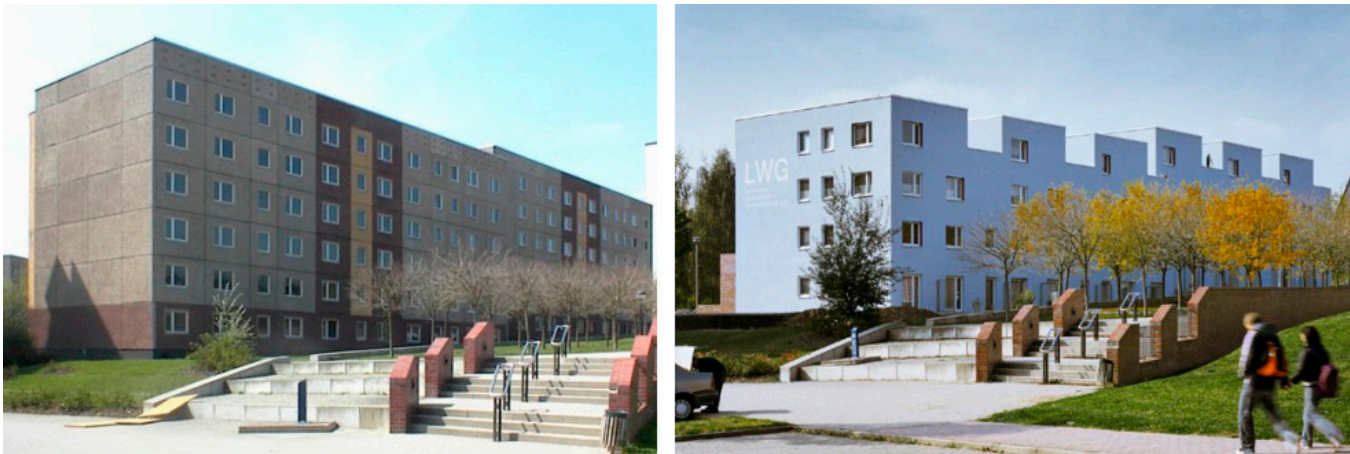
Figure 2. Transformation (selective demolition), Leinfelde residential building (source https://www.sfa.de/en/projekte/haus-06/ (accessed on 27 March 2024)).
