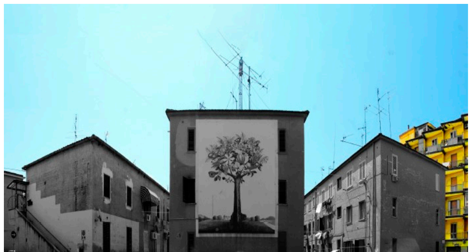
Figure 9. Current view of the residential complex.
