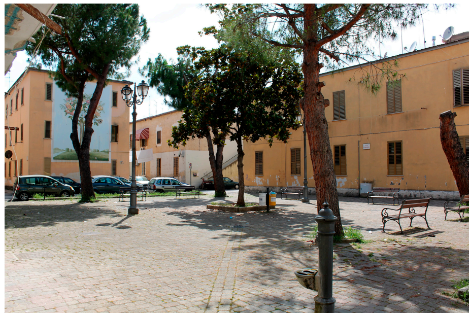
Figure 18. Actual photo of the building under study.
