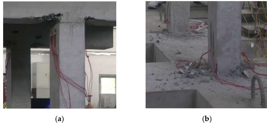
Figure 7. Column failure under the ordinary model: (a) column top destruction; (b) column bottom damage.
