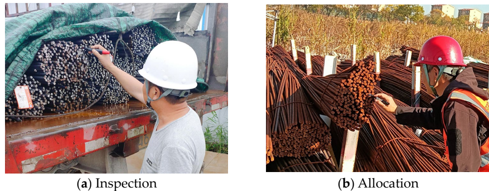
Figure 1. Manual counting of rebars.
