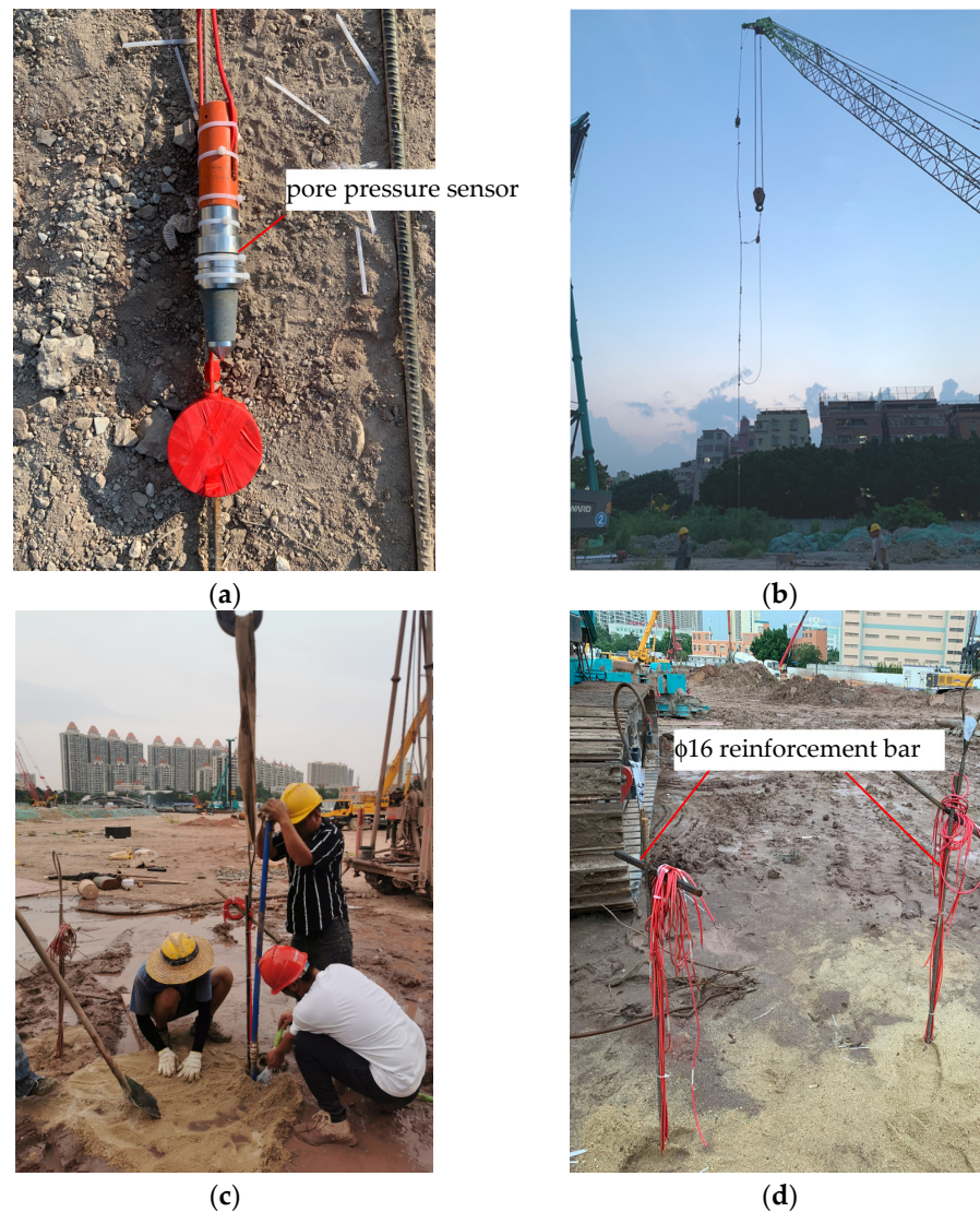
Figure 5. Pre-buried of pore pressure sensor: (a) securing the pore pressure sensor, (b) inserting the reinforcement bar and sensor, (c) packing fine sand and bentonite balls, and (d) burying the pore pressure sensors along with the reinforcement bar.
