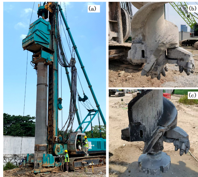
Figure 1. Construction equipment of DPC pipe piles: (a) pile driving equipment, (b) paddle-reaming bit 1, and (c) paddle-reaming bit 2.
