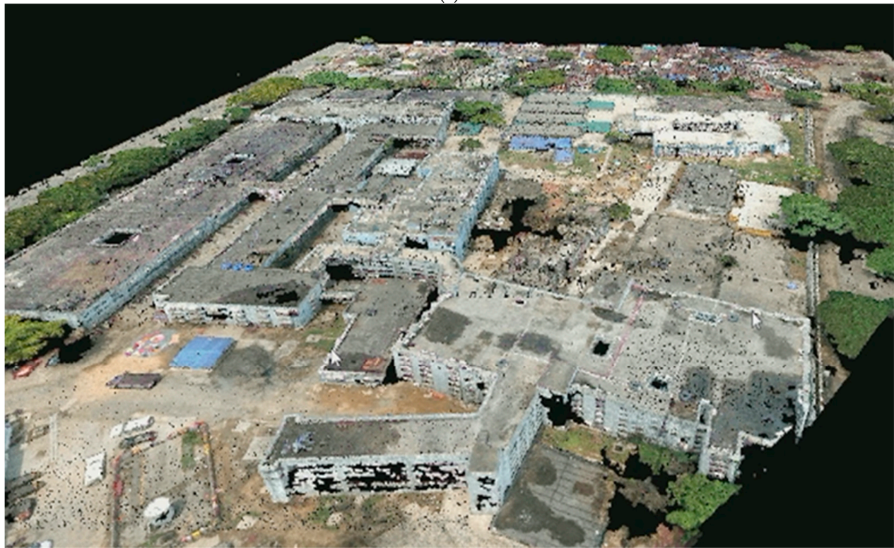
Figure 4. Digital surface models. (a) DTM RGB point cloud data showing the terrain elevation information. (b) The DSM point dense cloud shows all the features of the study area.
