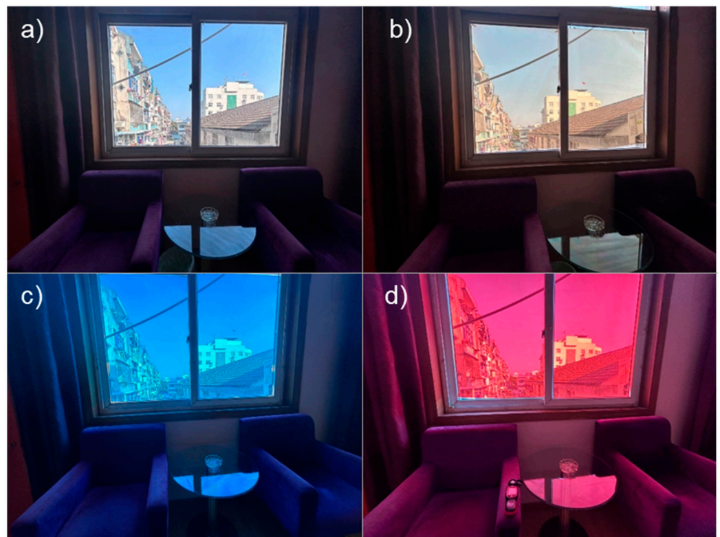
Figure 2. Four states of windows on lower floors: (a) clear (C2), (b) bronze (BZ2), (c) blue (BL2), and (d) red (R2).
