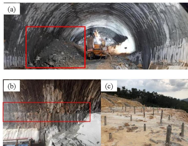
Figure 17. The emergency control measures: (a) backfill of debris in the tunnel; (b) spillway pipe at left arch of tunnel; (c) grouting at ground surface.
