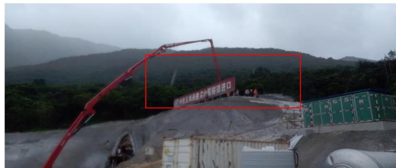
Figure 14. Grouting mortar at the top ground of tunnel.
