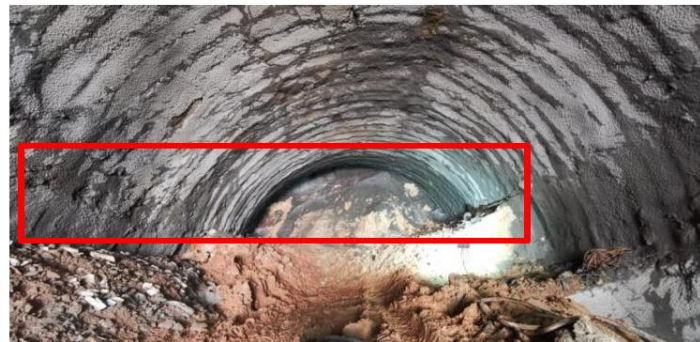
Figure 3. Tunnel surrounding rock deformation diagram.
