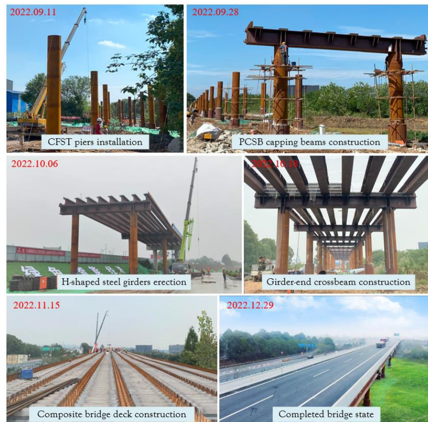
Figure 20. The onsite construction process of the Pengshan Qinglong Bridge.
