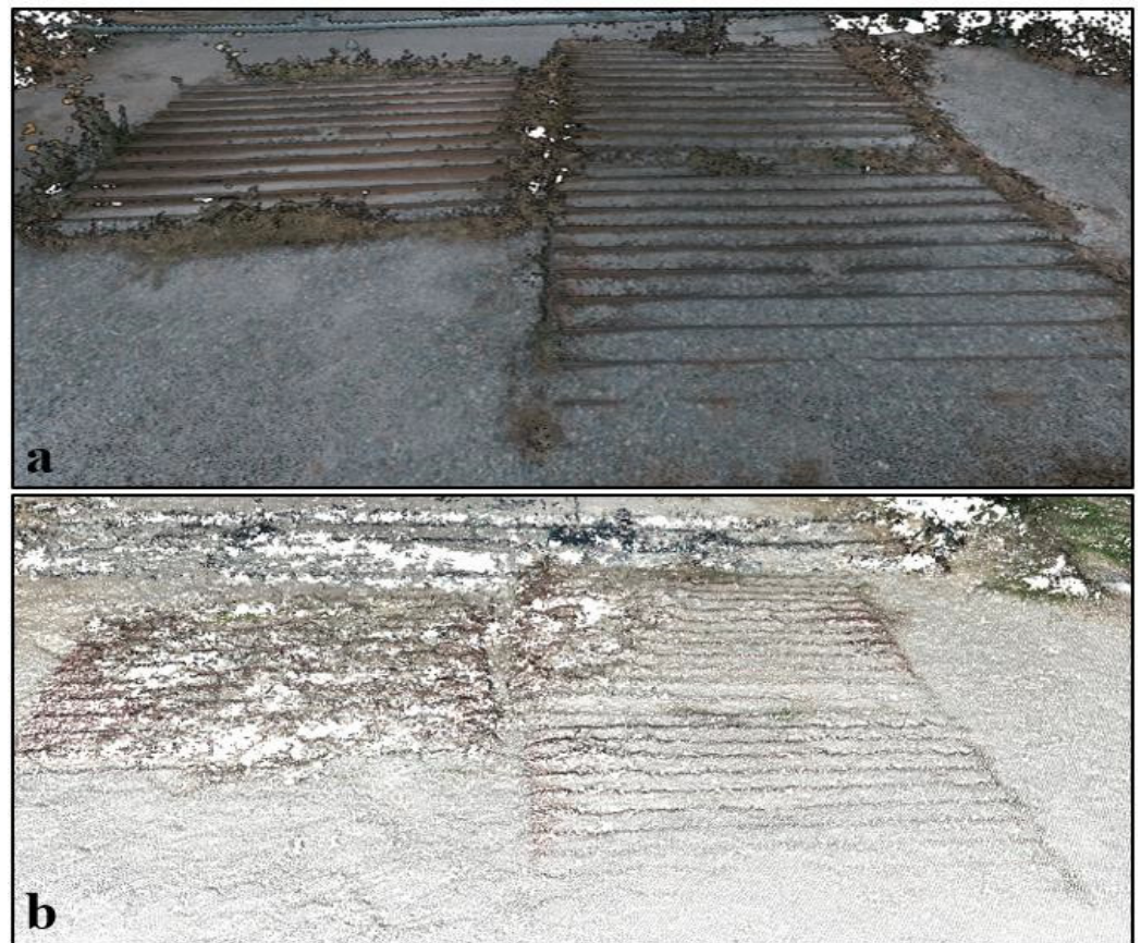
Figure 11. Lakeside north gate grating captured with the (a) Looq scanner and (b) DJI Air2S drone.
