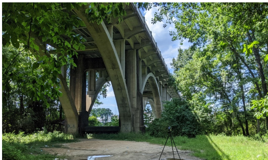
Figure 7. Dense vegetation around the bridge.
