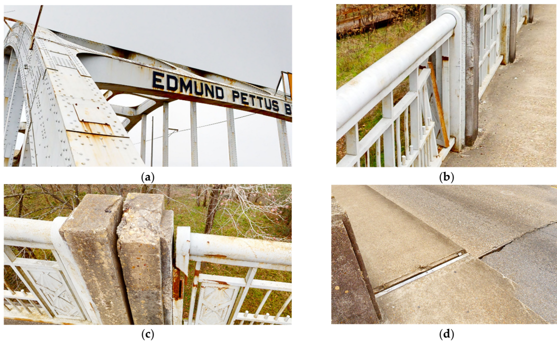
Figure 4. Places of the bridge needing maintenance and repairs. (a) Corrosion and paint maintenance needed along Span-2. (b) Damaged railing plate and baluster on Span-8. (c) Chipped and damaged cast-in-place concrete stanchion and broken baluster on Span-7. (d) Damaged expansion joint and missing cover plate near the north approach ramp.
