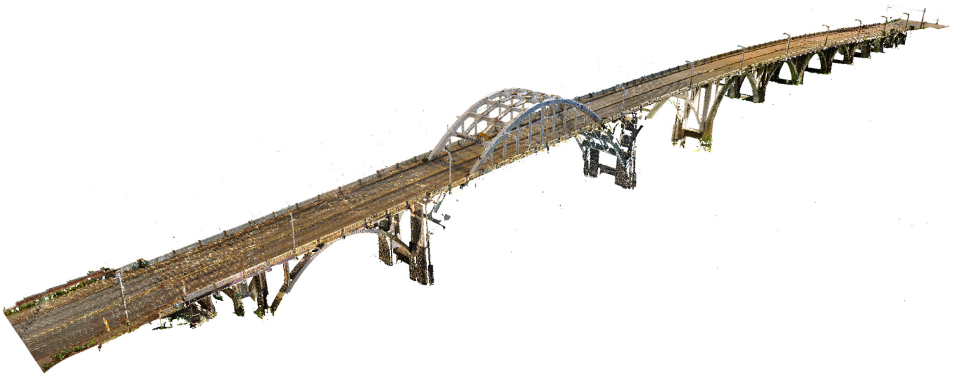
Figure 11. Registered point cloud of the whole bridge.
