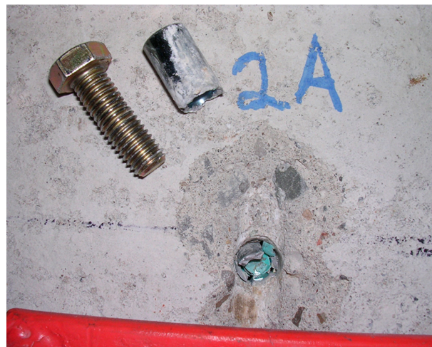
Figure 16. View of the 12.7 mm diameter anchor shear failure and concrete pry-out after ultimate shear test.
