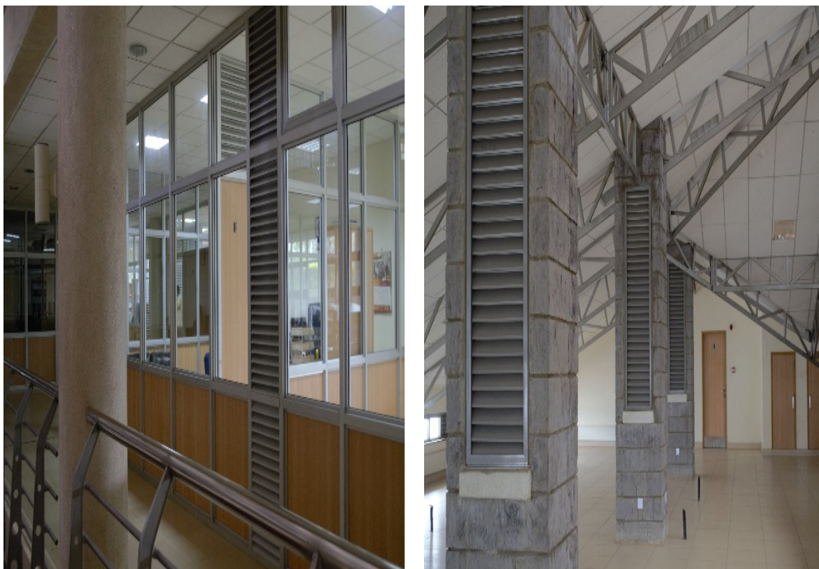
Figure 10. Louvered panels and exhaust chimneys, LRC. Source: Author 2023.
