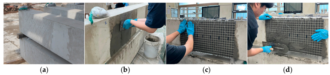
Figure 4. Strengthening methods. (a) Surface cleanup; (b) apply 1st matrix; (c) attaching textile grid; (d) apply 2nd matrix.
