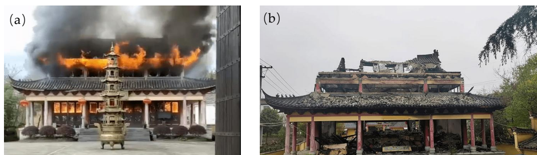
Figure 1. Shakyamuni Hall of Yanlong Temple. (a) Real fire scene. (b) Building scene after fire.
