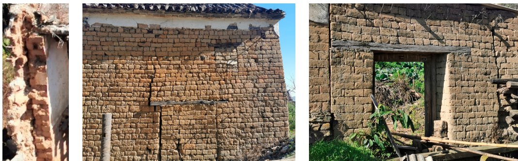
Figure 16. Adobe Brick Wall.
