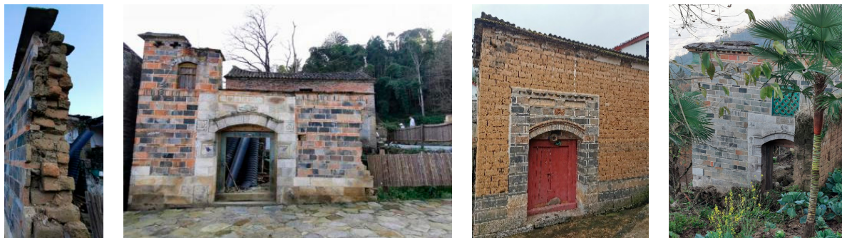
Figure 17. Hybrid Brick-Earth Wall.
