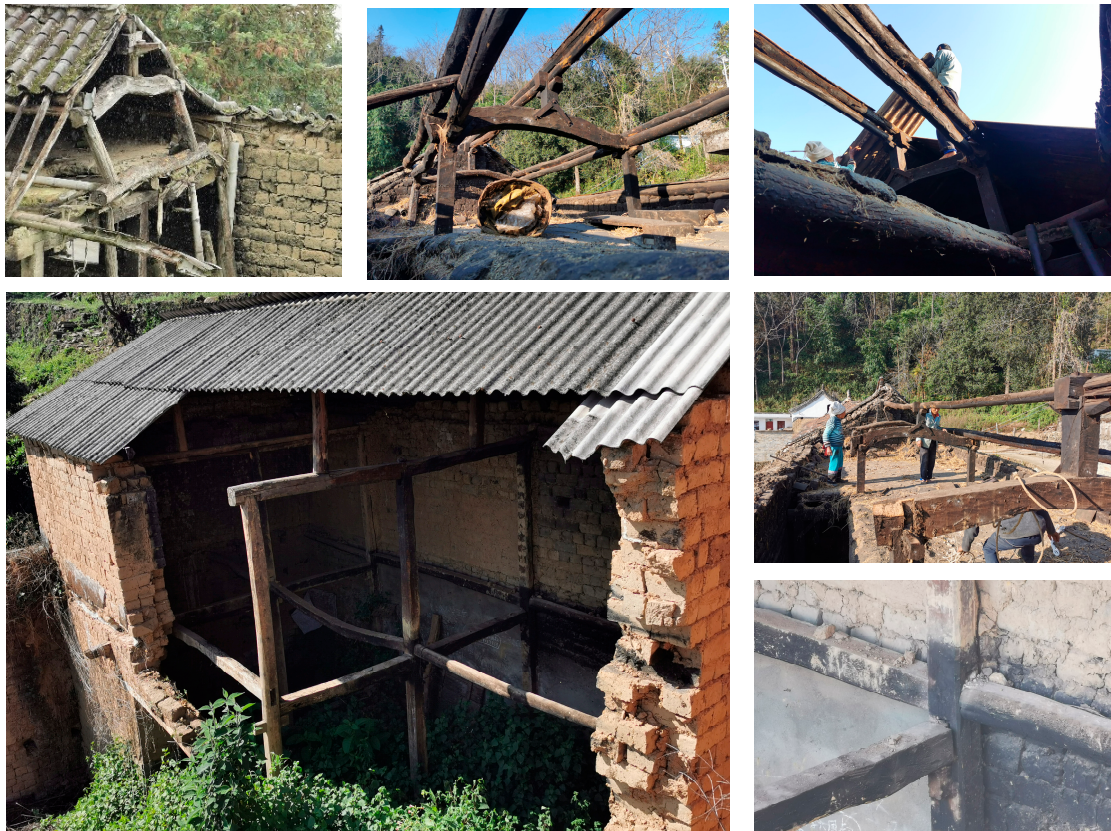
Figure 14. In-situ Documentation of Principal Wing Timber Framing Systems.
