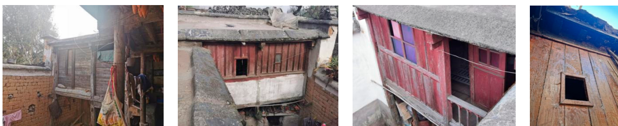
Figure 18. Timber Plank Walls.
