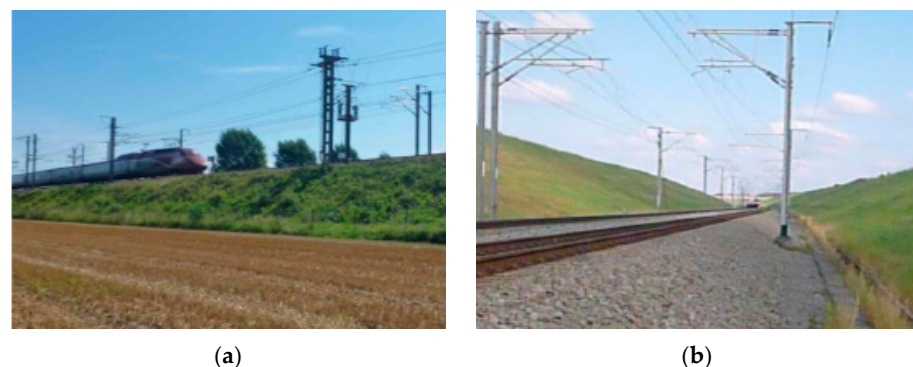
Figure 1. Test sections of the HSR: (a) embankment; (b) cutting.
