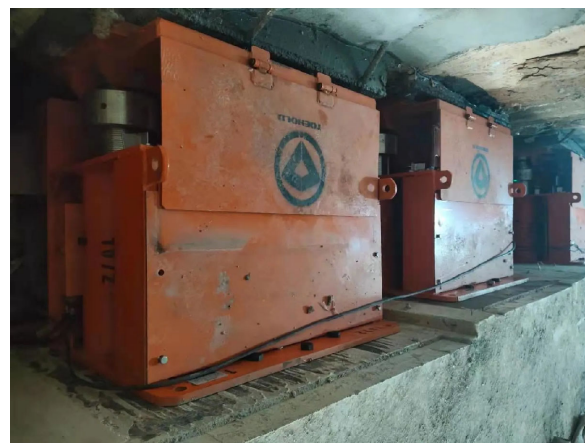
Figure 3. Servo steel strut system.
