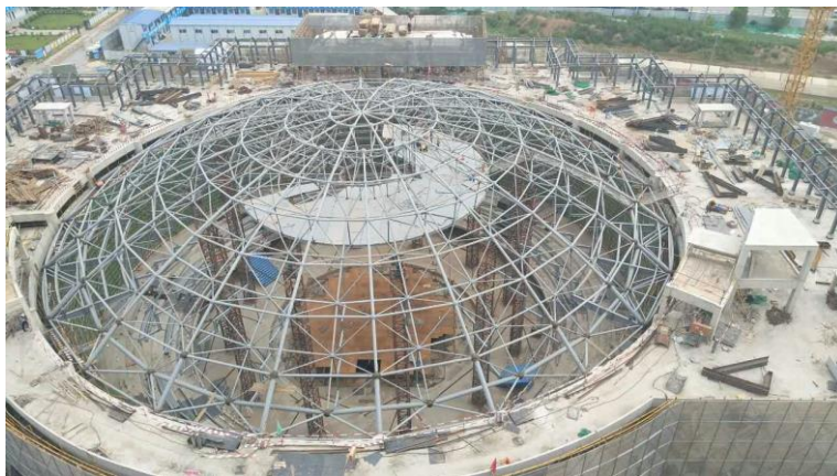
(a) Photo of completed steel space frame installation
