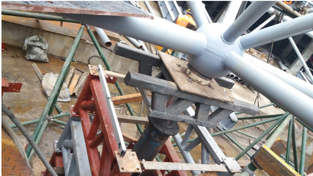
Figure 9. Field photograph of the support point during jacking.
