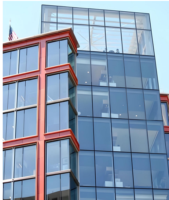
Figure 4. Glass curtain wall.
