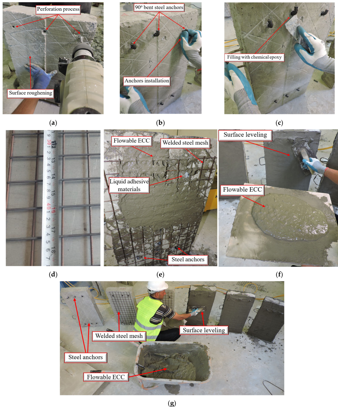
Figure 4. Strengthening of the samples: (a) surface adapting, (b) installation of steel anchors, (c) epoxy application for anchors, (d) the used welded steel mesh, (e) strengthening elements, (f) the used flowable ECC and (g) surface leveling.
