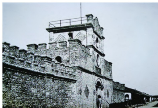
Figure 11. Clock Tower of the Tonghai Reclamation (Image Source: Reference [29]).
