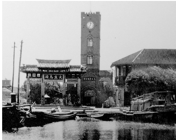
Figure 3. Clock tower at the Wharf of Dasheng No. 1 Spinning Mill, Tangzha, Nantong, Republican Era (Image source: Nantong Museum).
