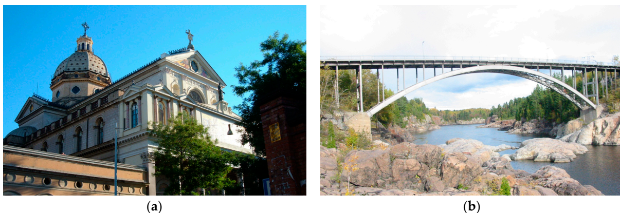
Figure 1. Early applications of aluminium in construction: (a) Dome of San Gioacchino in Prati, Rome, one of the first uses of aluminium in architecture; (b) Arvida Bridge, Quebec, the world's first all-aluminium long-span arch bridge [4].
