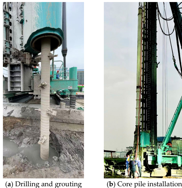
Figure 3. Construction process of PGP piles.
