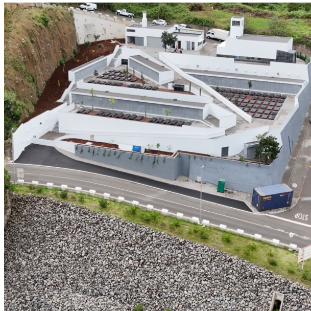
Figure 1. Panoramic view of the Porto da Cruz slope, illustrating the spatial interdependence between the cemetery (crest), the Regional Road ER110 (toe), and the Junçal Stream. The image highlights the high exposure to hydraulic erosion and the steep geomorphology typical of Madeira's northern coast (Source: Photographic survey adapted from CMM technical reports).
