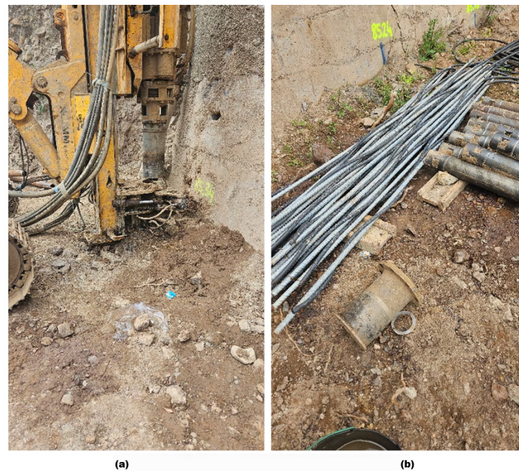
Figure 6. Execution of the 26 m micropile system. (a) Drilling operations in restricted spaces; (b) Handling of drilling equipment adjacent to existing structures. The design prioritized subsurface bypass over surface aesthetics to ensure structural stability (Source: Photographic survey adapted from CMM technical reports).
