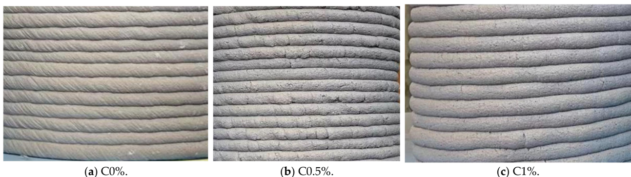
Figure 10. Extrudability assessment of 3DPC mixes incorporating different levels of OCS.
