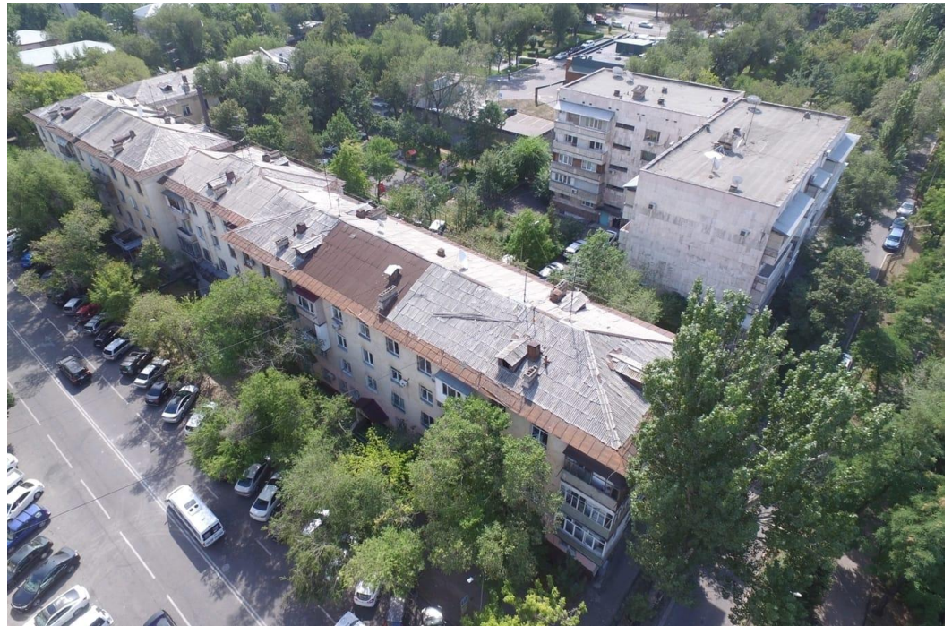
Figure 1. Four-story building with load-bearing brick walls.
