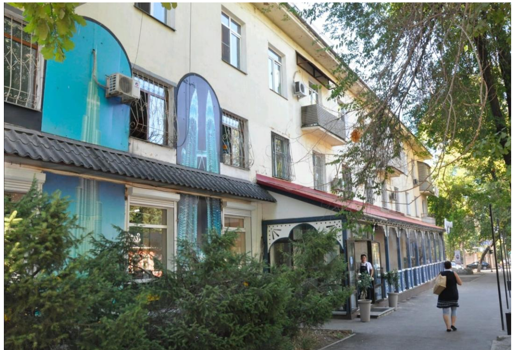
Figure 2. A three-story building with load-bearing brick walls.
