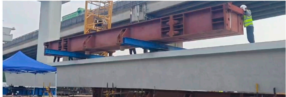
(a) Full-scale thin-walled box girder field photos
