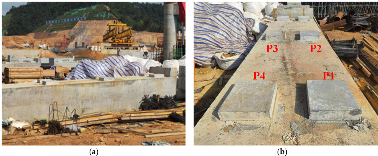
Figure 5. Field validation experiment at an ongoing bridge construction site in Zhaoqing City, Guangdong Province, China. (a) Overview of the construction site showing cap beam. (b) Close-up view of the cap beam and four cast-in-place concrete bearing pads (P1–P4), each with dimensions of 500 mm \times 500 mm.
